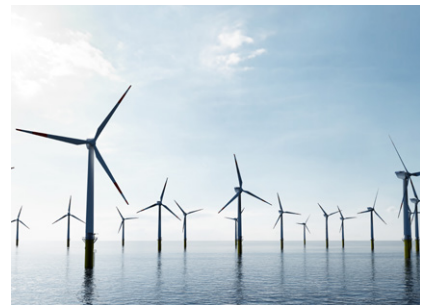
Offshore Wind Farm
